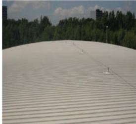
The roof before Solacoat was applied. The ambient temperature was only 28°C and the roof temperature was 57.2°C.
