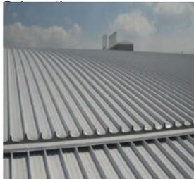
The roof after Solacoat was applied. The ambient temperature is 28°C and the roof temperature is now at 34°C.
